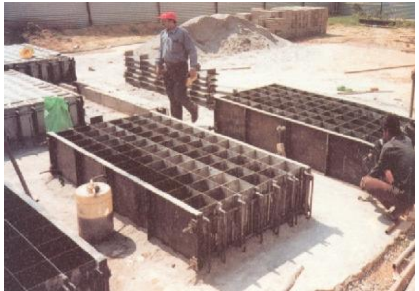
Light-weight block-production on site in India. Specially designed molds produced locally to Neopors specifications are assembled and waxed and poured with CLC density 1.000 kg/m 3 .
