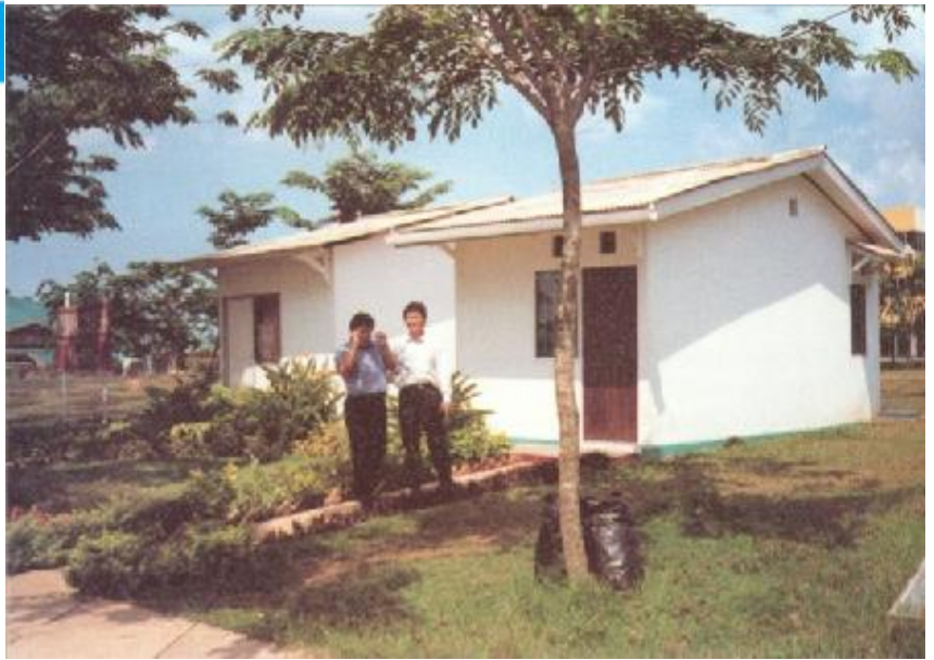
Affordable houses cast in-situ in Indonesia in density 1.200 kg/m 3 and wall-thickness of only 60 mm. One house each day per each mold. Frames for openings (d/w) and facility tubes cast-in.
