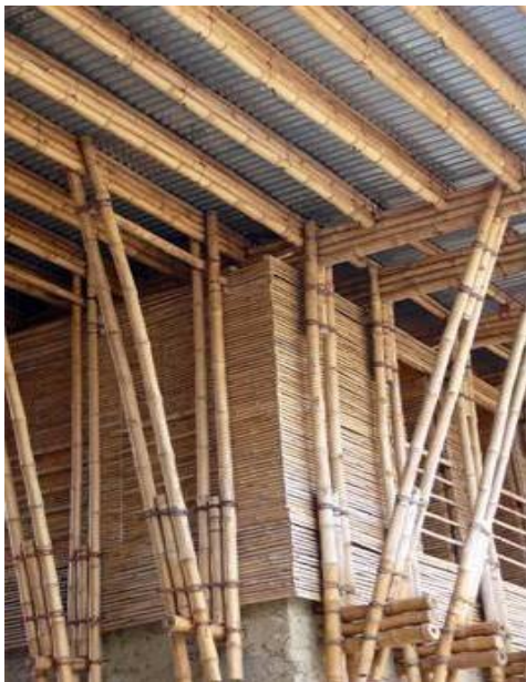
Left: Innovative bamboo framing at the Handmade School.
