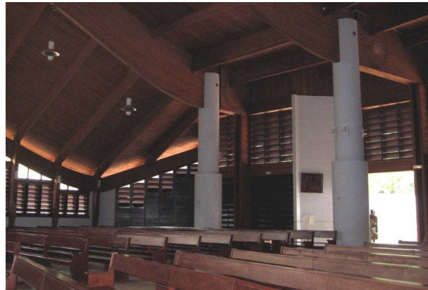
Below: Breezy wood louvers in a Yaounde, Cameroon church.
