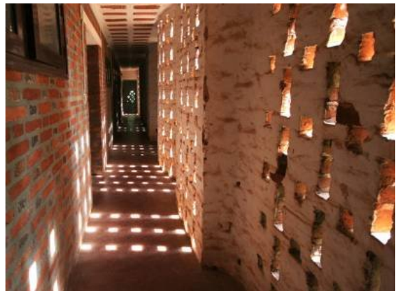
Above: A corridor defined by a brick screen or jali, by Sri Laurie Baker.
