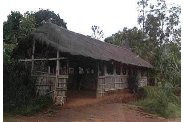
Above: An old reed and thatch building in Cameroon.
